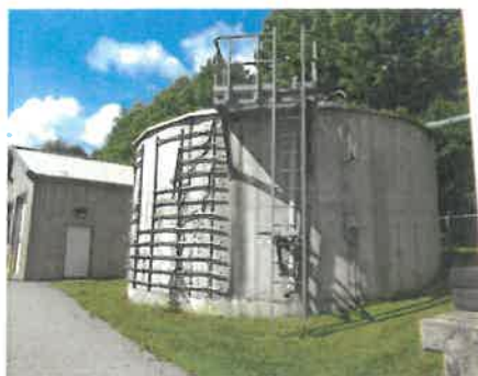
Aerated Sludge Storage Tank No. 2
