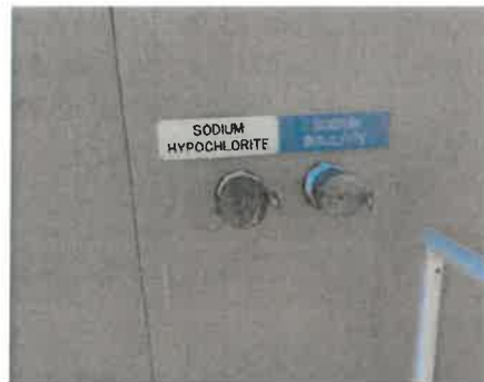
Truck Unloading Station
