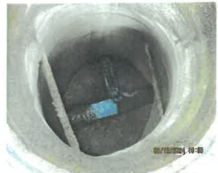
No ID – Wall + Water St.
