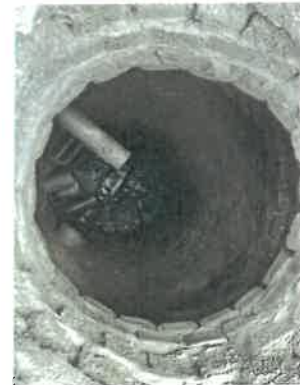
No ID – Next to NU Parking Lot
