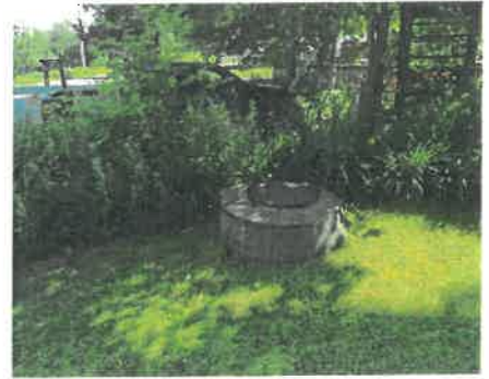
Pump Station Manhole
