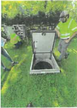
Pump Station Pit
