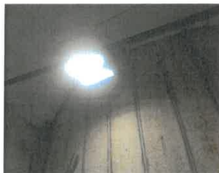
Aerated Sludge Storage Tank No. 1 Inside Garage
