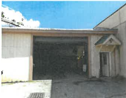
Control Building Entrance
