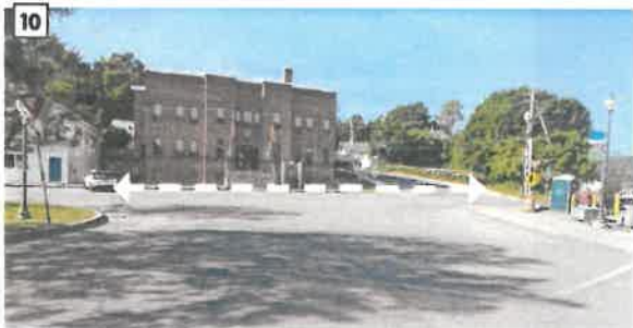
The crossing at Depot Square is 88 feet, and driver's approaching this intersection may be distracted as they look for parking.
