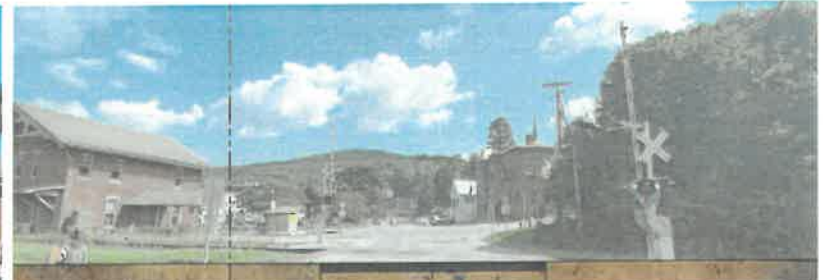
Image above: the existing railroad, without an official pedestrian crossing. Image below: section of the proposed solution.
