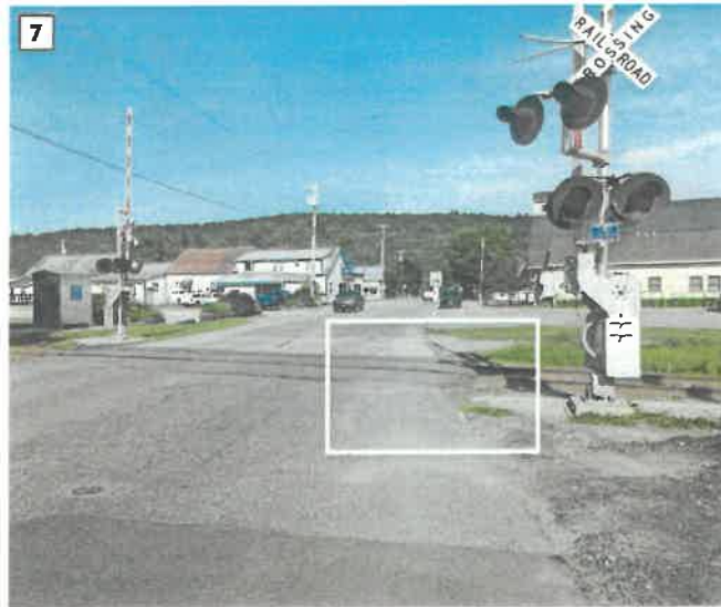
There is no formal pedestrian crossing at the intersection of the train tracks and Wall Street
