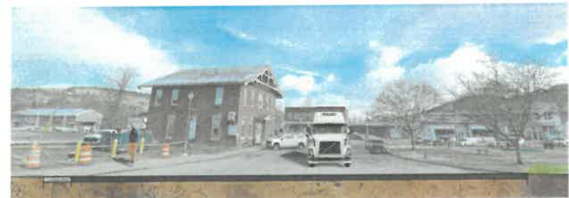
The existing crossing at Depot Square
