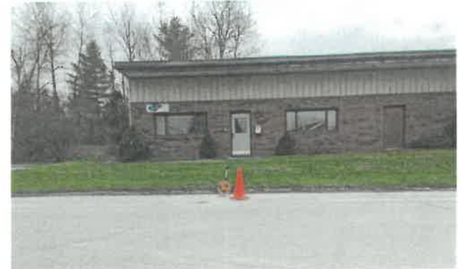
The new crosswalk location (noted by the traffic cone). By crossing in this location, pedestrians avoid the 52 foot driveway crossing at 173 Wall Street
