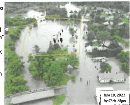
July 10, 2023 by Chris Alger Image of the 2023 flooding, partially mitigated by Dog River Park (called out in yellow.) Photo credit: Chris Alger
