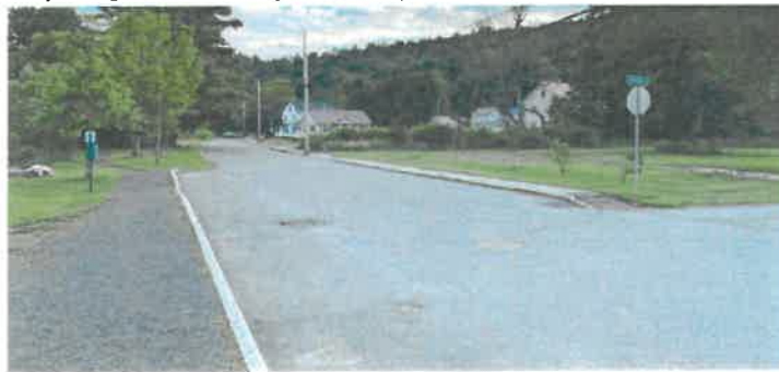
There is only one curb cut next to the Dog River Park parking area, and the landing area is not paved
