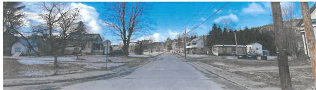
The existing sidewalk on Water Street's west side may make an additional sidewalk on the eastern side redundant
