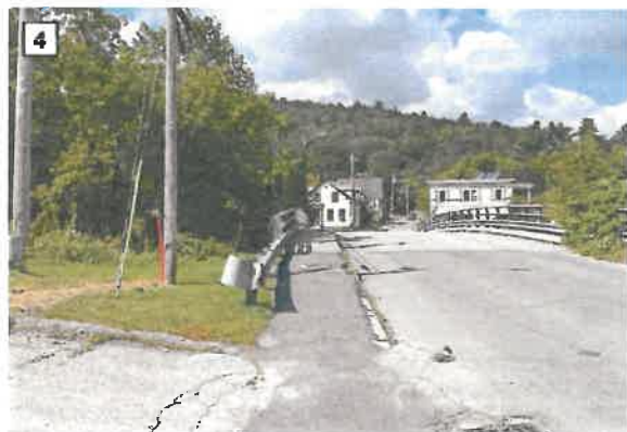
Existing sidewalk on the Wall Street Bridge
