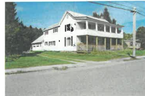
Property #4 362 Water Street
