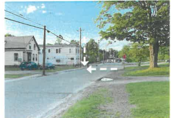
The current intersection of Wall and Water Streets lacks a defined crossing and a curb cut on Wall Street's west side. This design adds both.
